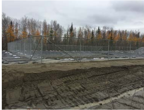
Construction of fenced detention basin
