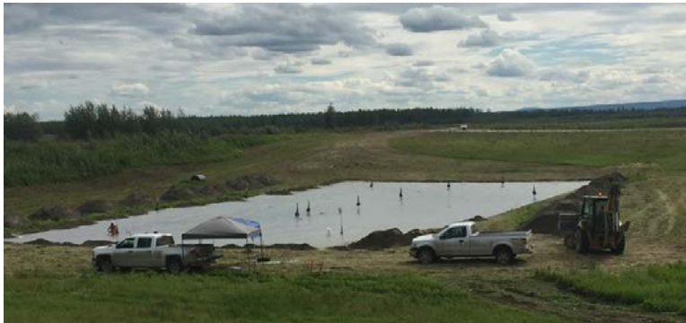
Installing bioventing cover at Site FT001
