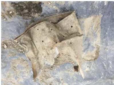
Drywell constructed of perforated 55-gallon drum
