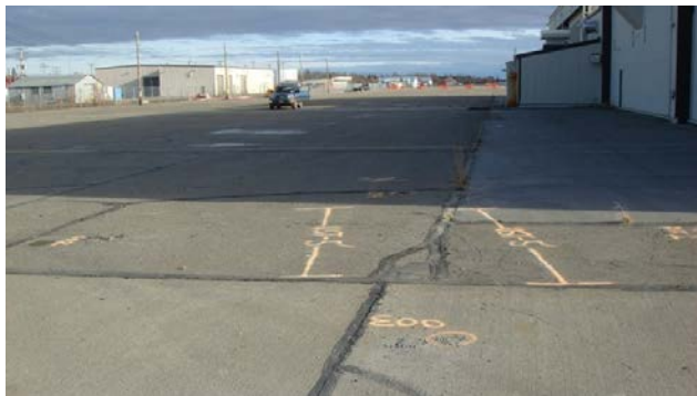
Northwest corner of CAC Building where USTs were formerly located.
