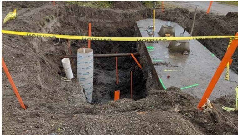
Excavation area around former fill stand
