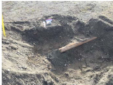
Plugged Pipe at OAP under runway
