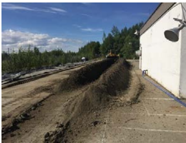
Tilling soil at Missile Storage Yard
