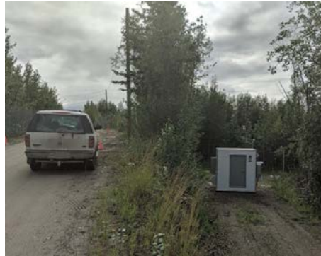
Blower enclosure building for air sparge system.
