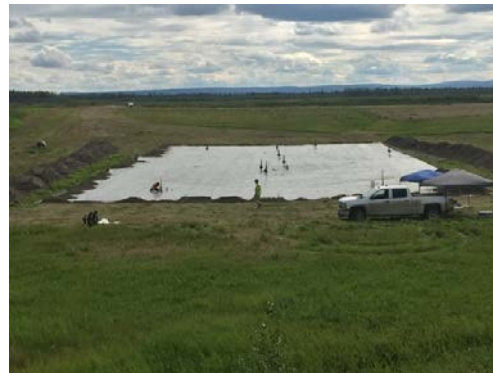
Installation of Bioventing Cover at Former Fire Training Protection Area (Site FT001)
