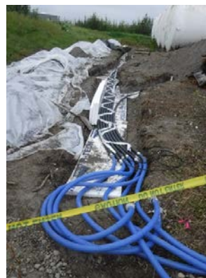
Installation of SVE piping
