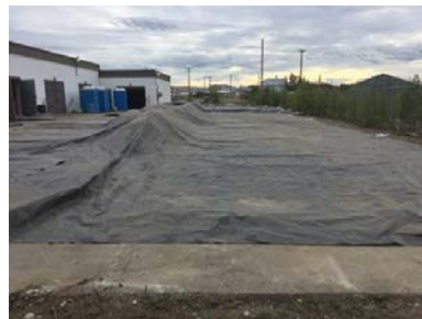
Soil covered pending test results
