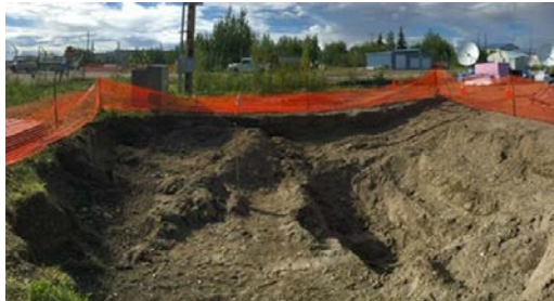
Excavation at Site CSS001
