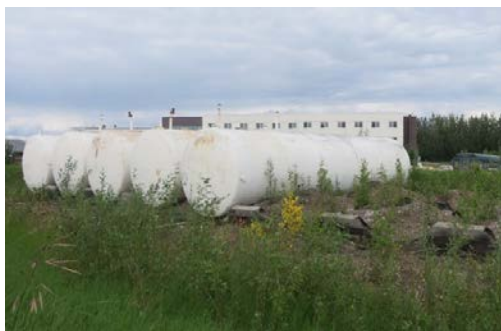
Tank farm ASTs at Site ST005 Area C
