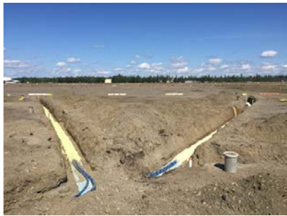
SVE vent pipe installation at Site SS015
