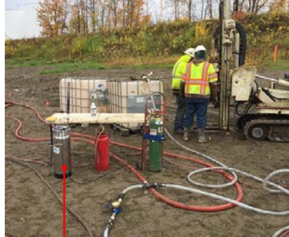
Injecting Bioaugmentation Culture
