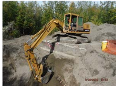
Excavation at Site CST013
